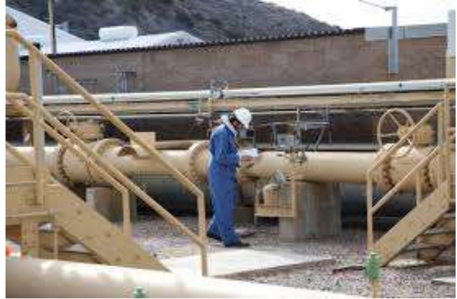
Source: SoCal Gas
